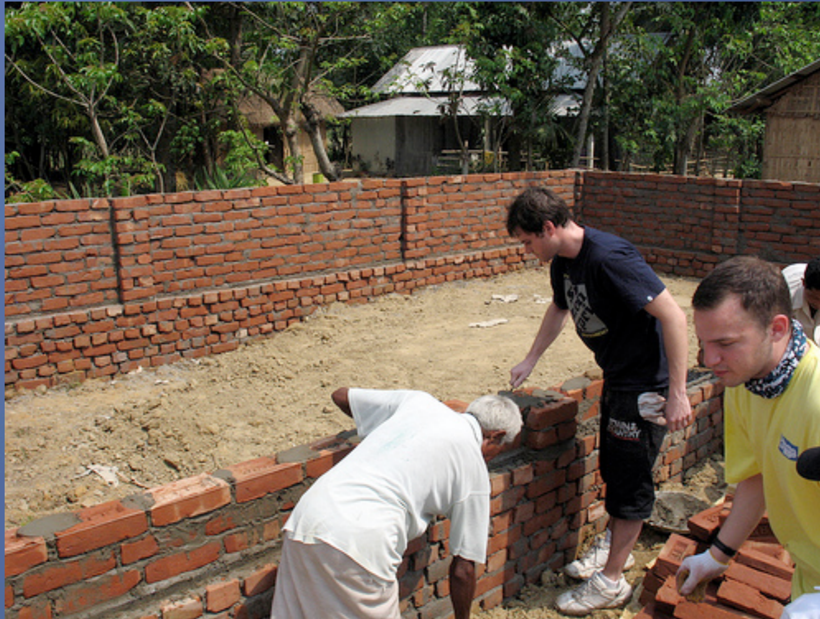
© Bricklaying by MC MasterChef via Flickr
